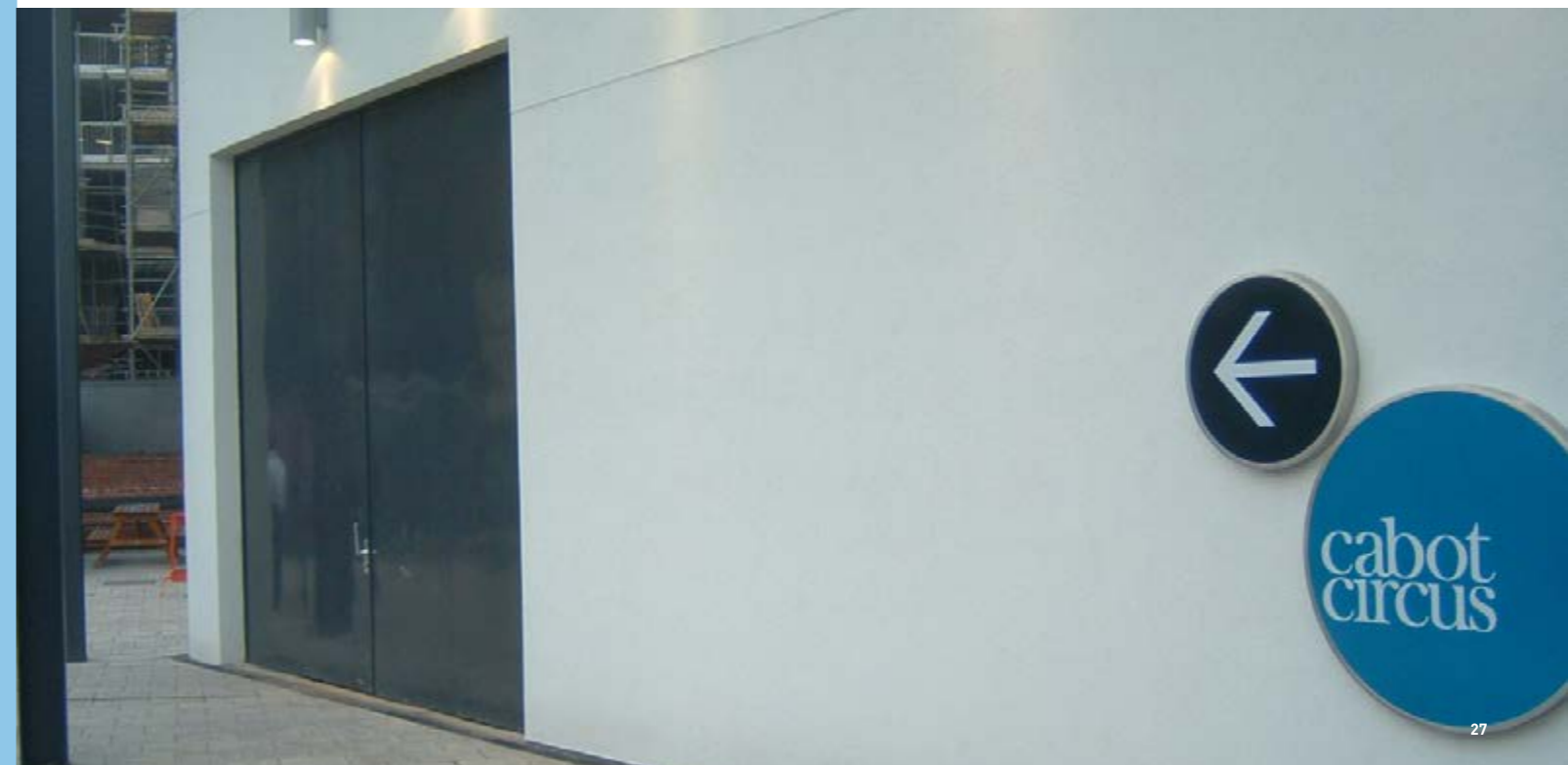
Cabot Circus Plant Room, Bristol
